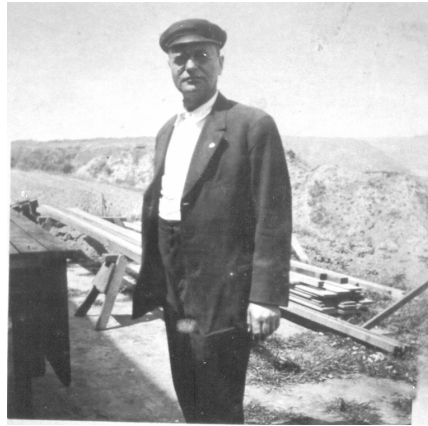
64. Mr Heindel during the building activities in 1913.
